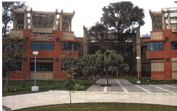
Figure 3.1: Front view of CESE, IIT, Kanpur
