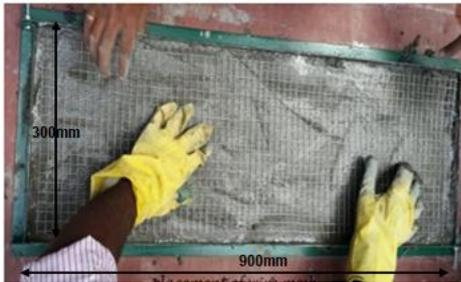
**Figure 2:** Fabrication of ferrocement panel
