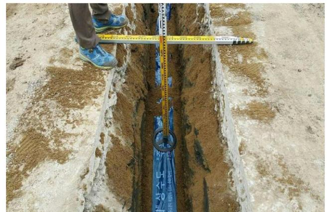
**Figure 5:** Measurement of the burial depth with a staff
