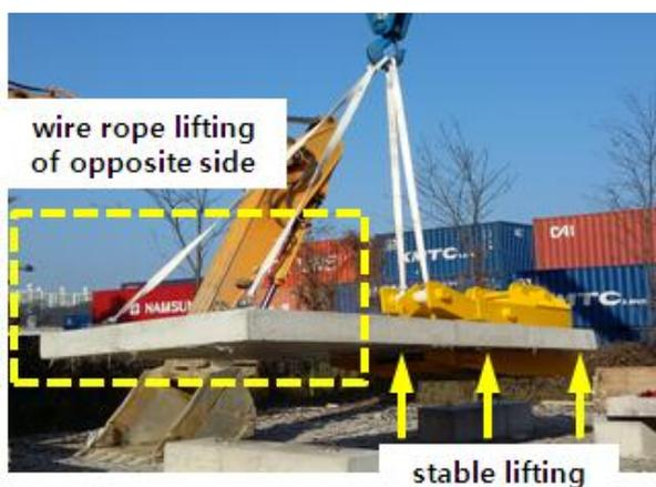
Figure 8. Test scene of bridge deck lifting using wire rope on the opposite side
