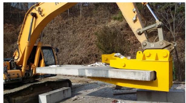
**Figure 6.** Test scene of concrete lifting using a 10W excavator
