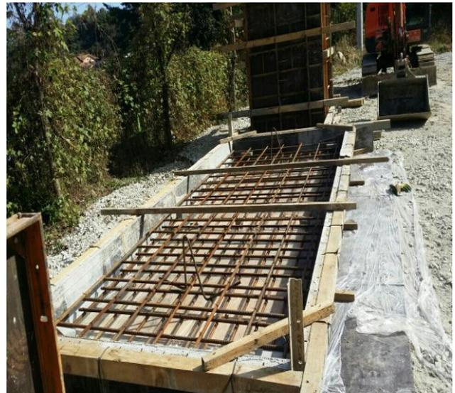
**Figure 5.** Test scene of concrete pier specimen
