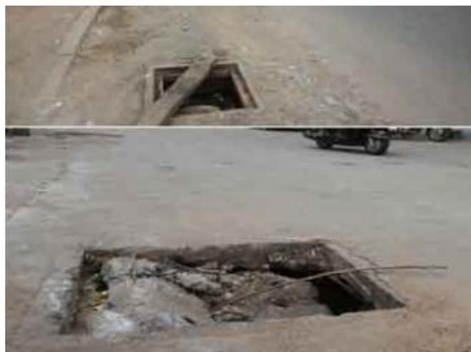
**Figure 3:** Improperly closed man-hole
