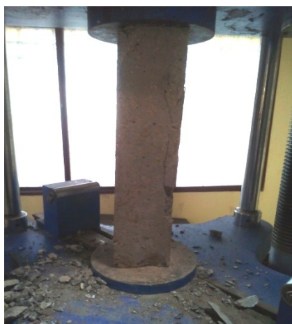
Figure 8. Crack pattern in Control Columns
