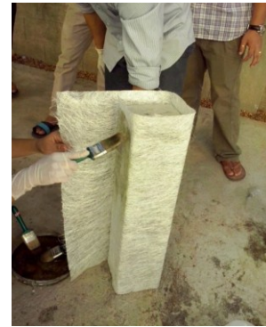
Figure 3. Wrapping of GFRP mat in Column
