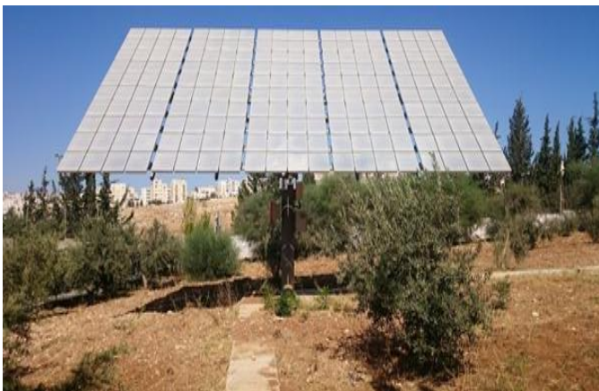
Figure 6: Sample of Applied Science Private University solar energy plant, Amman, Jordan, a (CPV)
