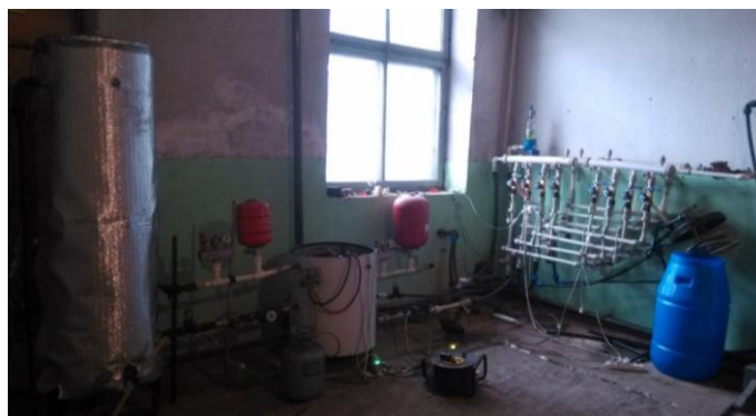
Figure 3: General view of the experimental stand
