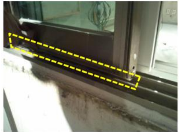
(b) The horizontal air-tight structure installed at vertical part
