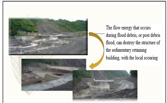
**Figure 1.** The process of local scouring on the downstream of sabo dam structures.
