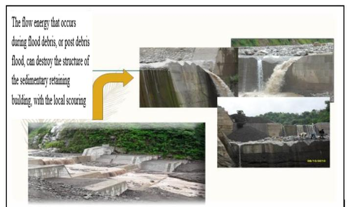
**Figure. 2.** The process of abrasion on downstream of Sabo dam structure.
