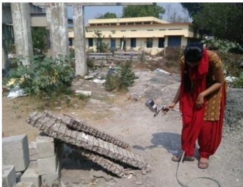
Fig. 3 Sand blasting of chipped beam
