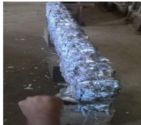
Fig.5 Applying epoxy resin
