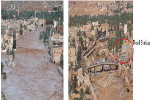
Figure 15: Area View Of The Overflow Of Wadi M'zab The Morning Of 9 th October 2008
