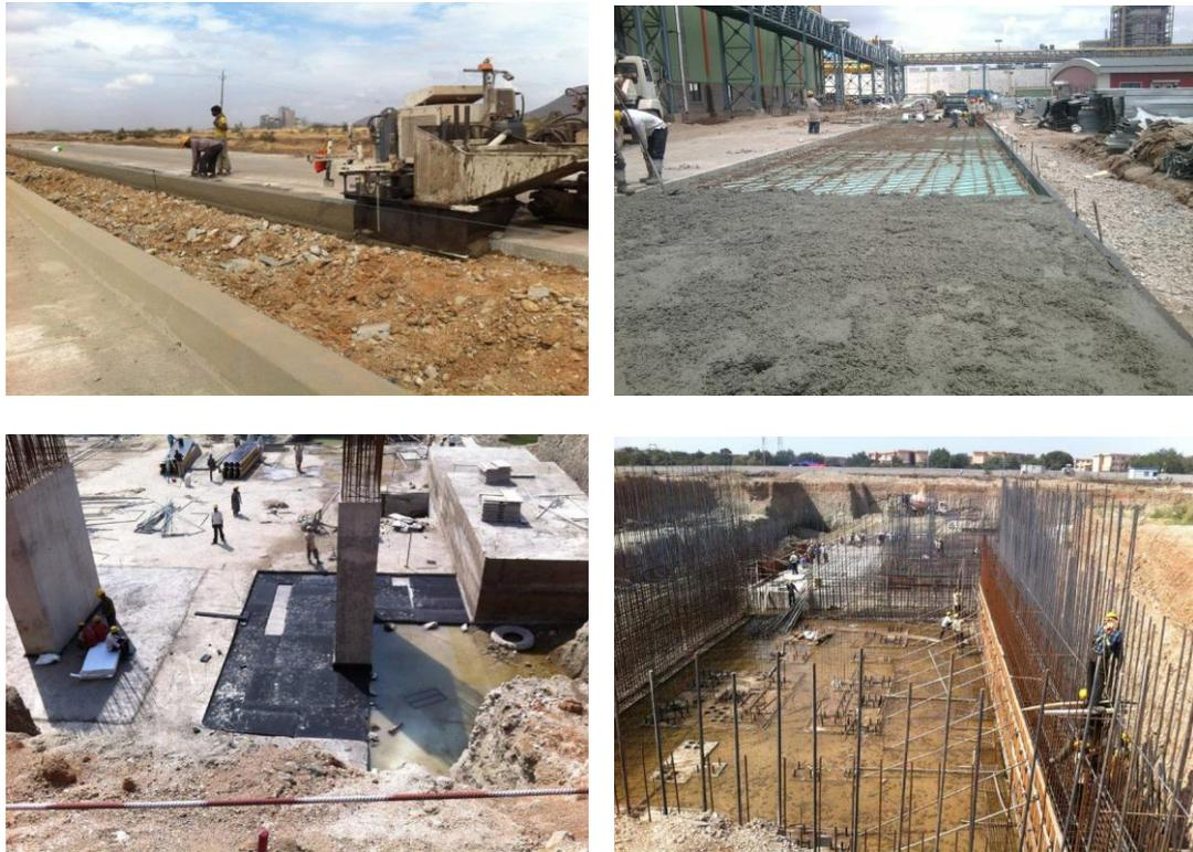
**Fig 11:** Usage of granulated BF slag and crusher dust at JSW Vijayanagar works
