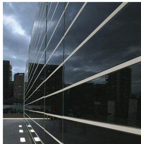
Solar PV Façade is aesthetically pleasing, generates electricity & helps in better energy performance of the building. Transparency in Solar PV Façade can be obtained by spacing between solar cells or see through thin film solar cells. Light effects can also create nice patterns on the same.[1,7,9]
