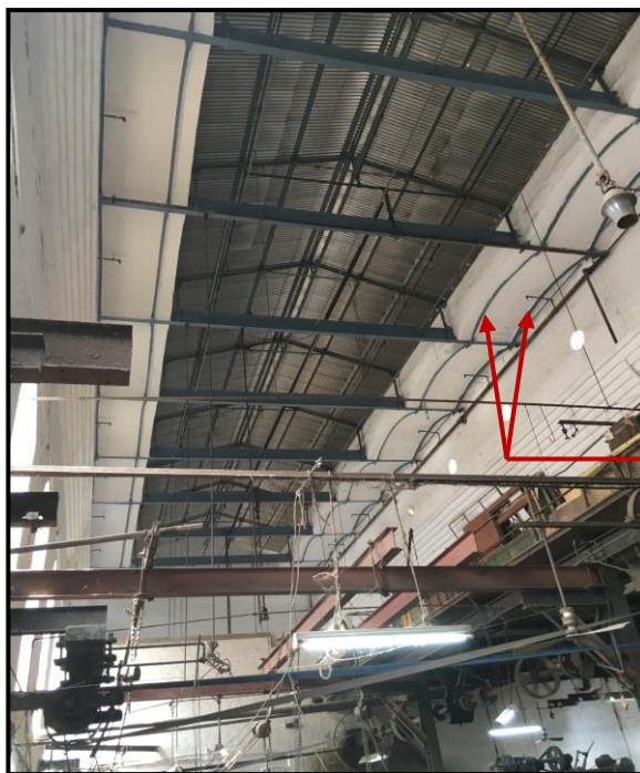
PLATE 6 : PHOTOGRAPH SHOWING STRENGTHENING OF JACK ARCH AT SOFFIT LEVEL BY ISA 50x50x6
