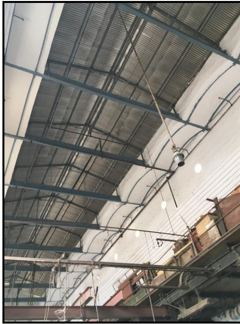
PLATE 5 : PHOTOGRAPH SHOWING CONDITION OF ROOF STRUCTURE AFTER REPAIR.
