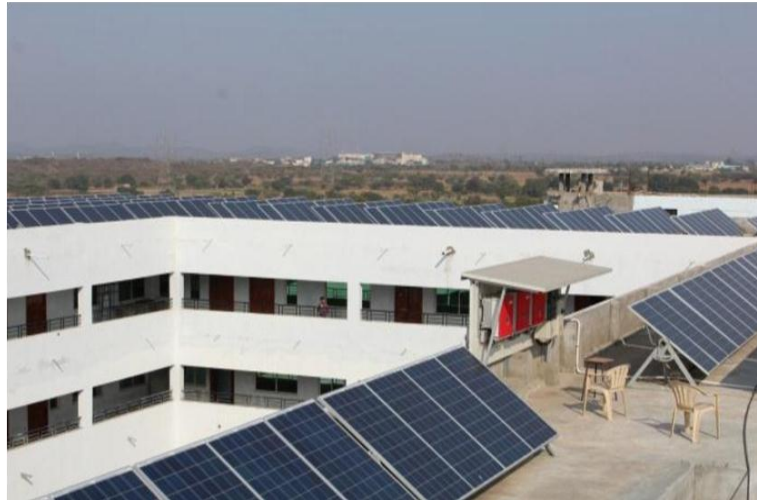
Fig. 2 120kW p Solar PV Plant on EEE Block of CVR College of Engineering
