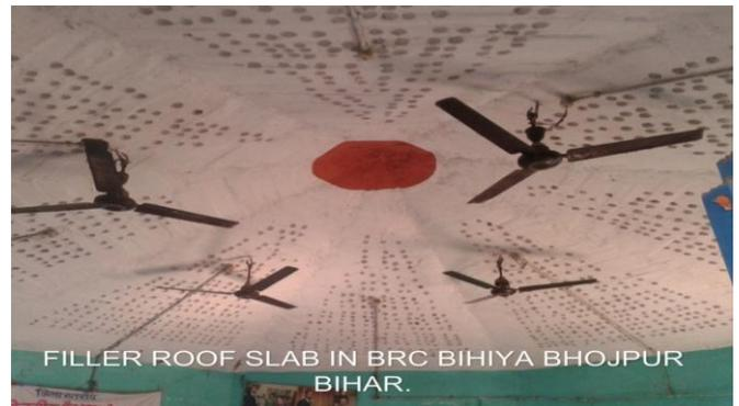
Fig.5: The use of filler slab in study area Block Resources Centre, Bihiya
